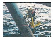
A one man lightweight staging system installed by rope access teams to provide a stable work platform for carrying out steelwork repairs/renewals, blasting and painting and other remedial work.
