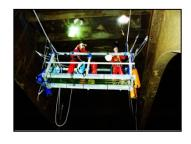
TOPCAT is a tailor made lightweight staging system that can be installed by rope access teams and, once in place, provides a stable working platform that enables one or more technicians to perform tasks such as blasting, coating repairs, steel repairs / renewals etc.
